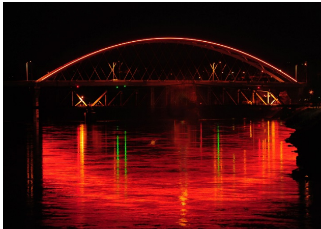
The Amelia Earhart Memorial Bridge in Atchison was lit in orange last year as part of National Work Zone Awareness Week.
